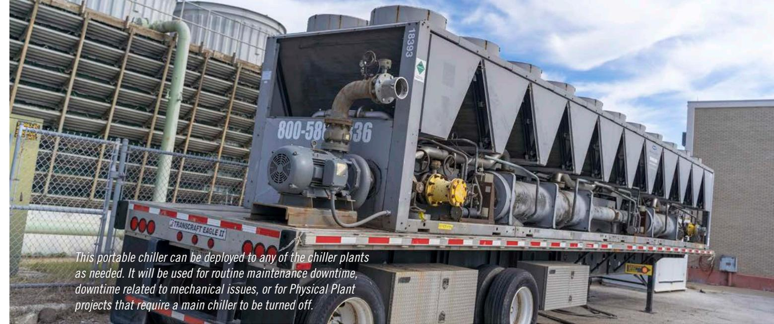
*This portable chiller can be deployed to any of the chiller plants as needed. It will be used for routine maintenance downtime, downtime related to mechanical issues, or for Physical Plant projects that require a main chiller to be turned off.*
