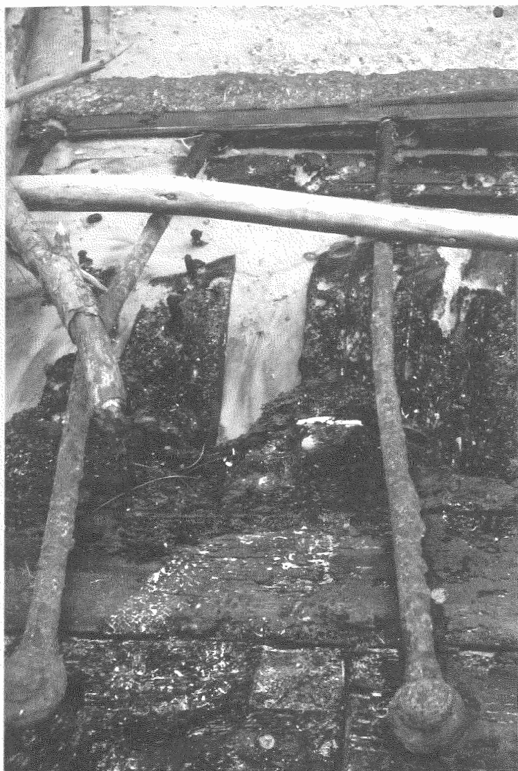
Figure 13. Two of the 5 remaining iron chains extend up from a piece of the chain wale, amid a tangle of tree branches; between them at bottom is a small rectangular patch, just below which are the heads of two spikes, of Muntz metal (left) and iron (right).
