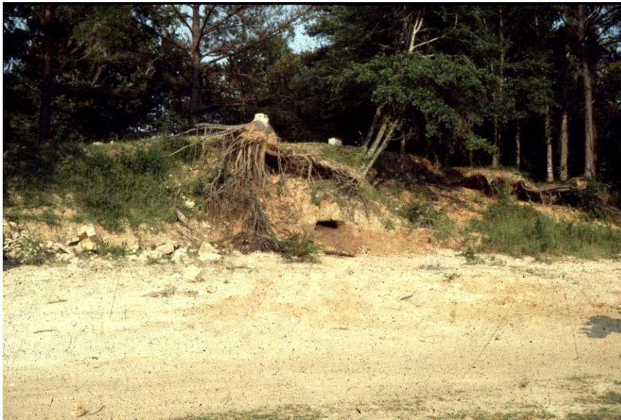
Figure 29. Chattahoochee Landing (8Gd4) Mound 2 in 1978, view facing southeast, from river side, showing looter excavation (black oval) tunneling into bottom slope, and heavy erosion undercutting trees.
