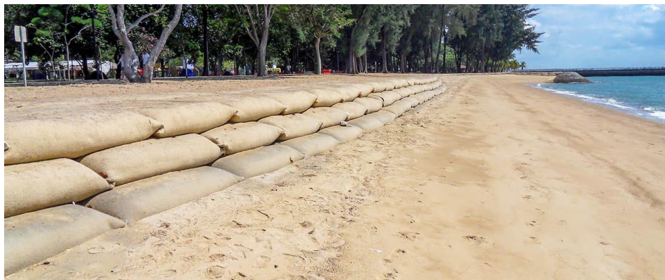
Figure 10. Geotextile Sandbags (SECUTEX®, 2019)
