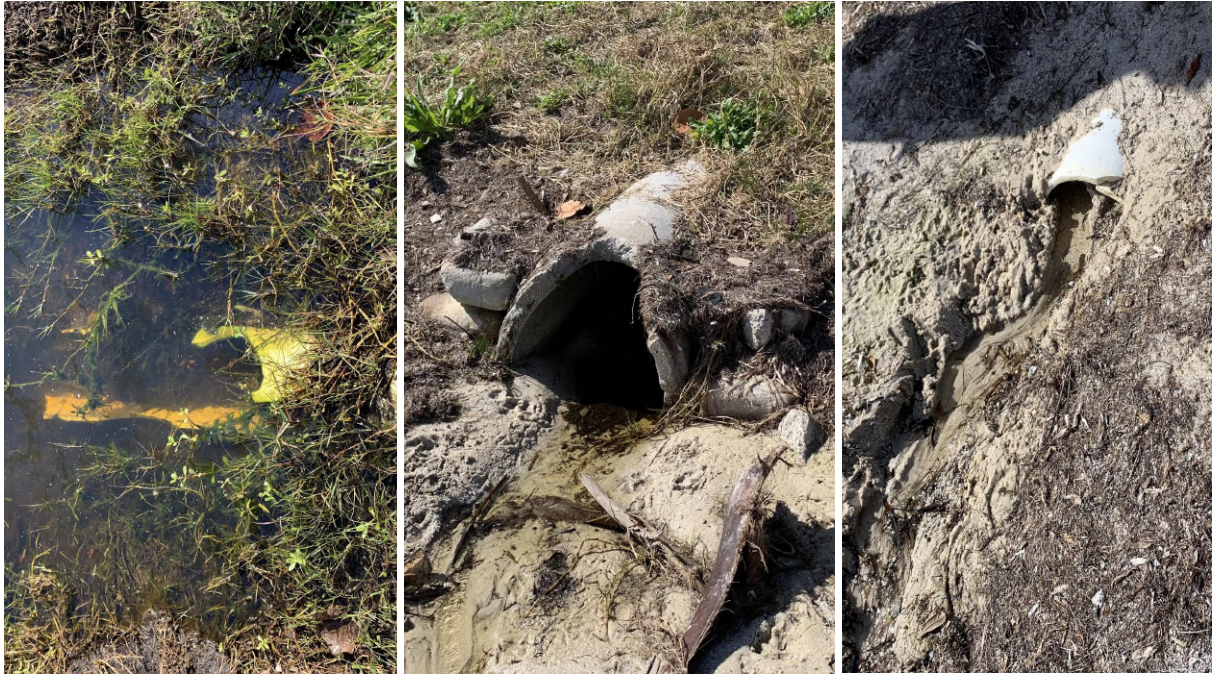
Figure 4. Existing Stormwater Piping in Poor Condition
